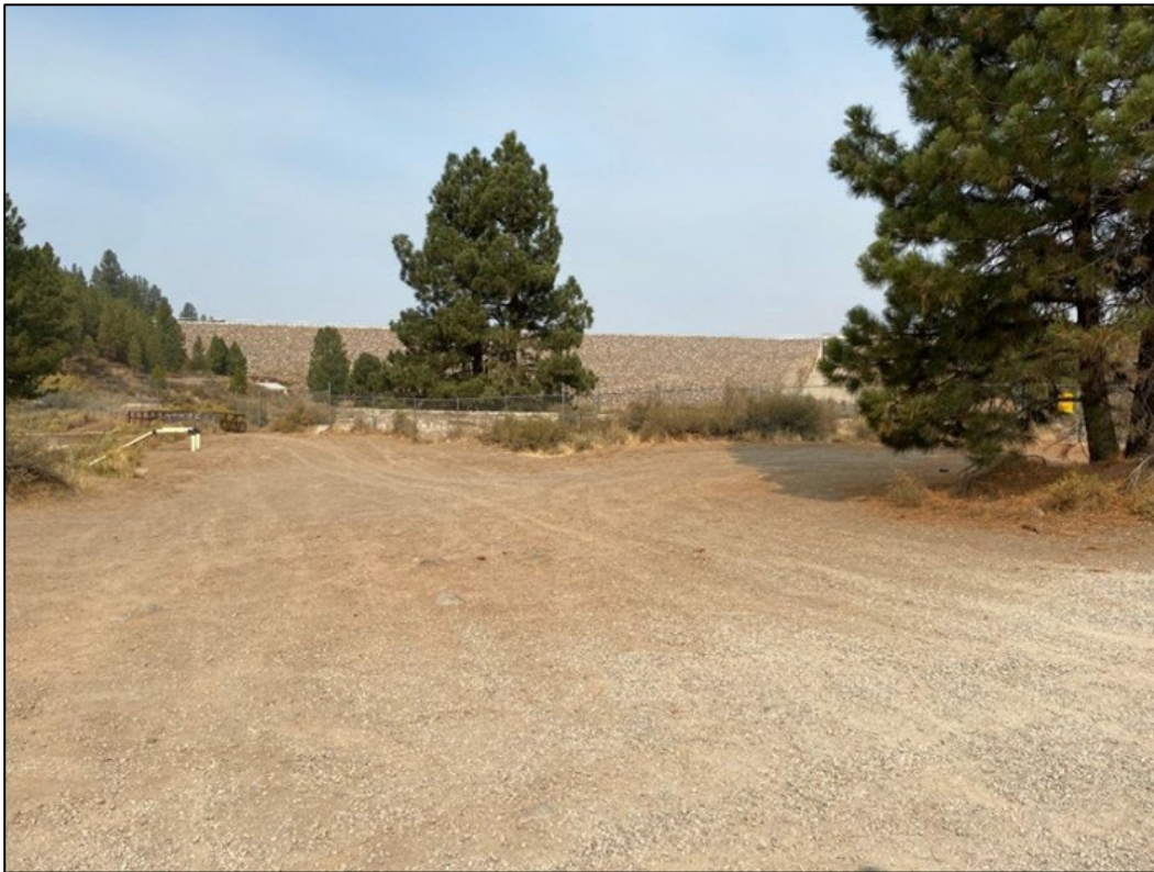
Photo 4. Boca Dam staging area looking northwest towards Boca Dam.
