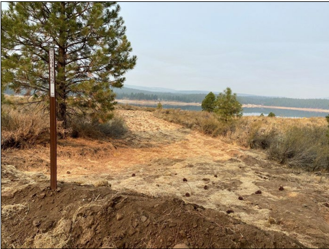
Photo 5. Example of a decommissioned road south of the Boca Reservoir.
